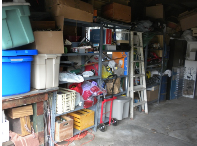
B3. Garage walls not visible
