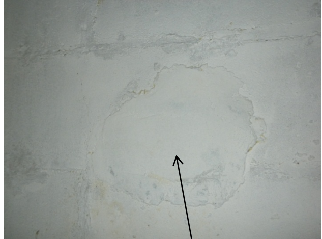
E3. Removed oil pipes
