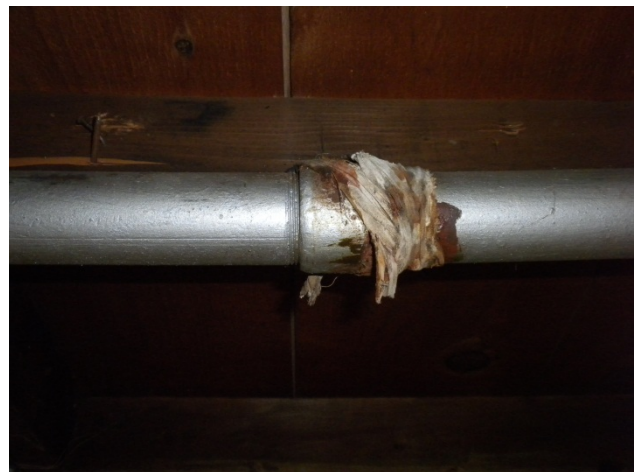
F1. Temporary pipe repair
