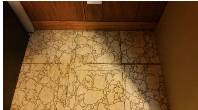
Water stained tiles east side
