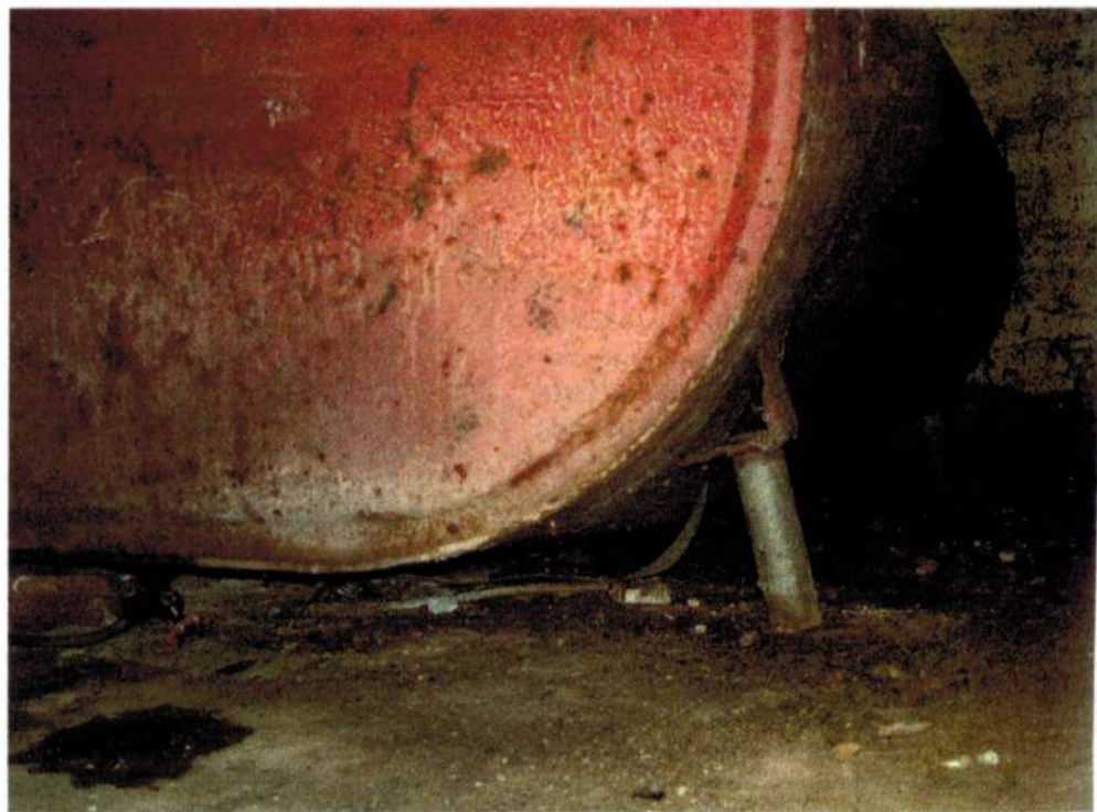
The result of a bad tank leg.
