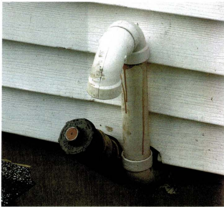
The vent pipe should be changed to steel pipe and a proper vent cap should be installed. The way this is now, it would be fairly easy for an insect nest to clog the vent.
