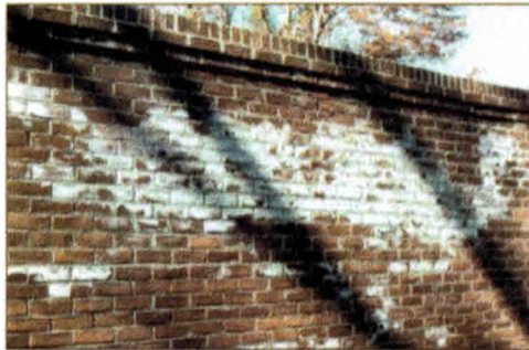
Photo 1, Efflorescence
