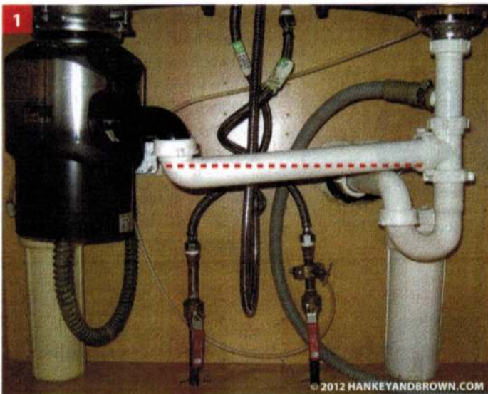
Photo 1 shows the improper slope of a disposal drain. The reverse slope of this drain will permit water and food waste particles to collect below the dashed red line. This improper slope increases the potential for clogging and foul odors.
