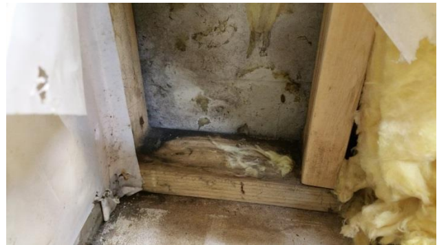
Wall & floor water stains
