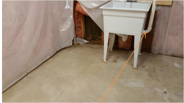
Improperly vented standpipe
