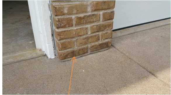
Brick veneer supported on driveway
