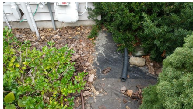
Short exterior sump pump discharge pipe
