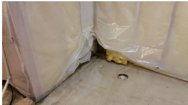
Water damaged wood & insulation
