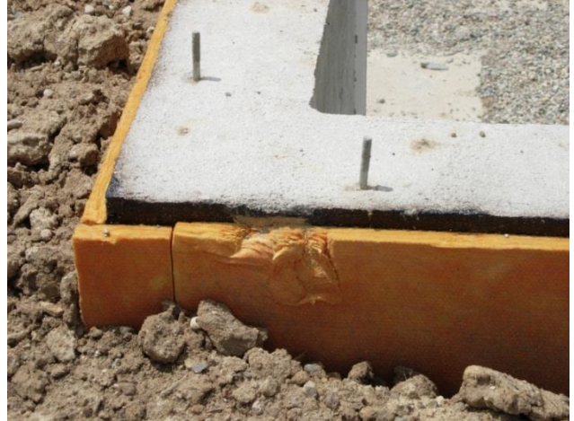
1 st inspection foundation insulation
