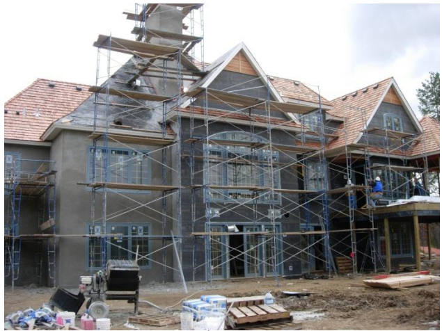
3 rd inspection exterior barriers
