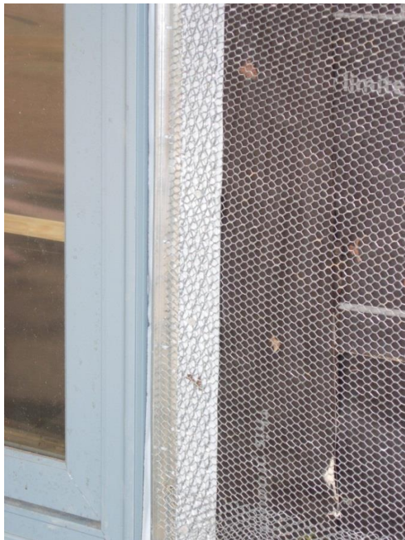
3 rd inspection flashing
