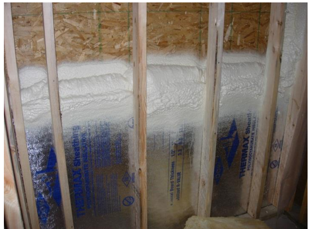
3 rd inspection insulation
