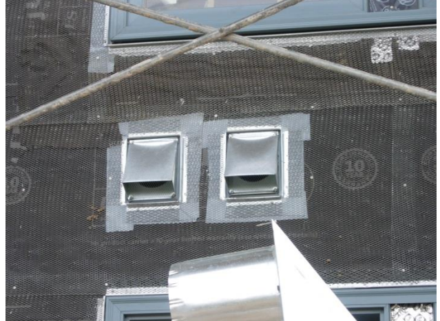
3 rd inspection flashing
