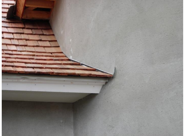
2 nd inspection flashing
