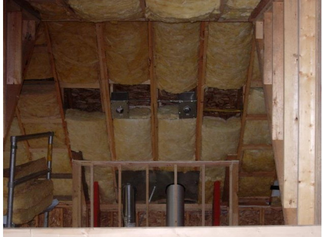
3 rd inspection vaulted ceilings
