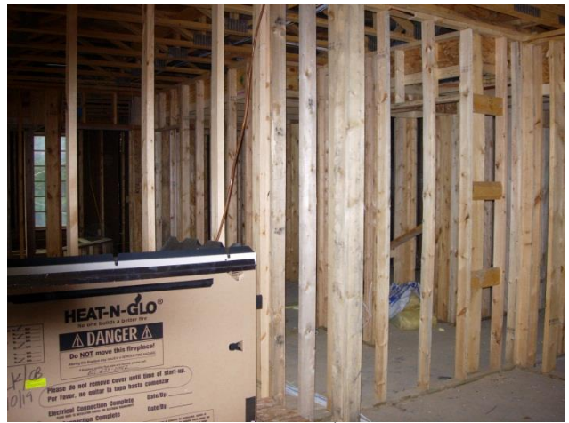
3 rd inspection basement
