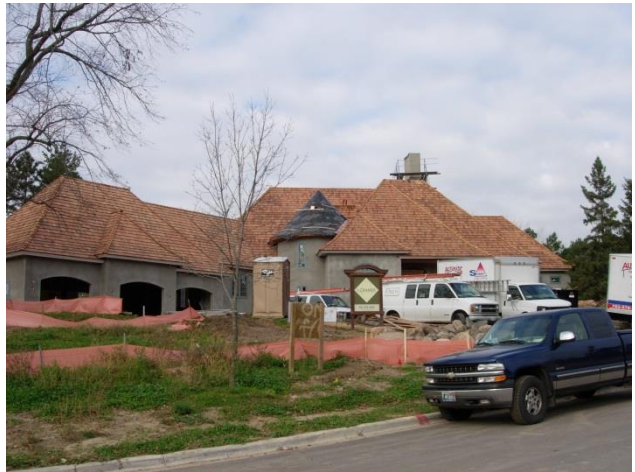
2 nd inspection building framing
