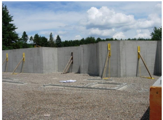
1 st inspection backfill & wall bracing
