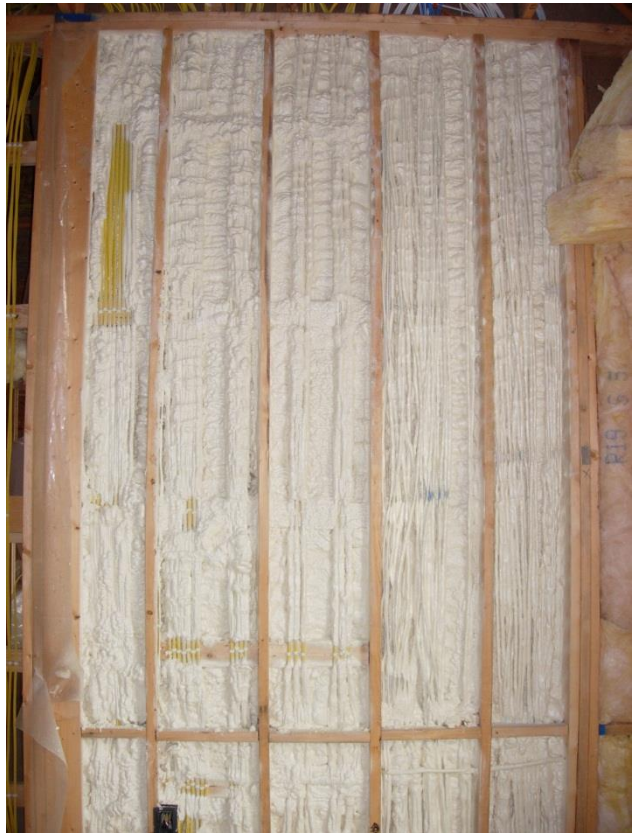
3 rd inspection insulation
