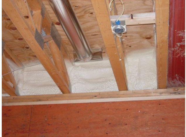
3 rd inspection insulation
