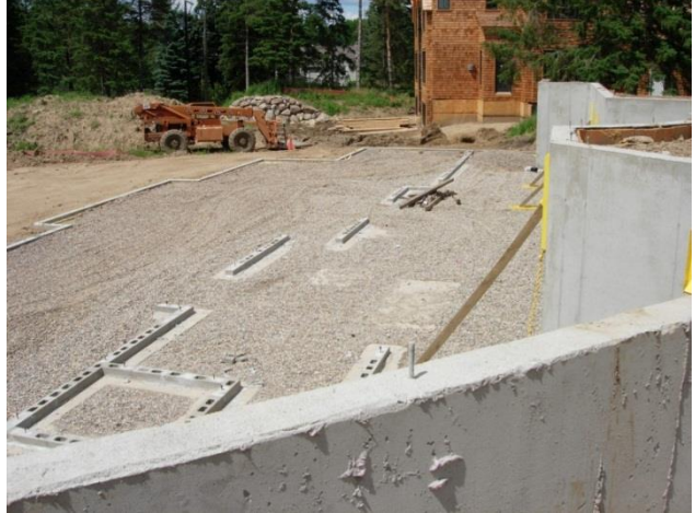
1 st inspection interior footings
