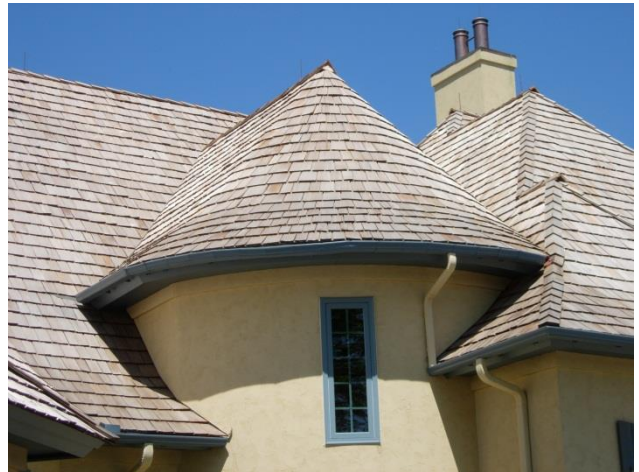
4 th final inspection
