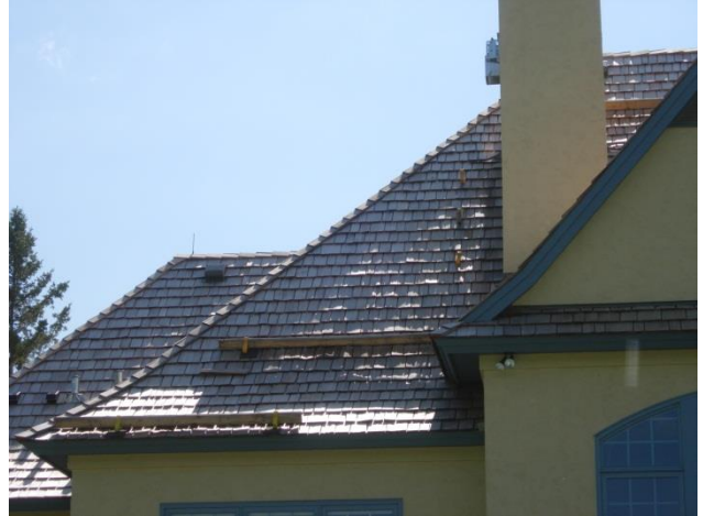
4 th final inspection
