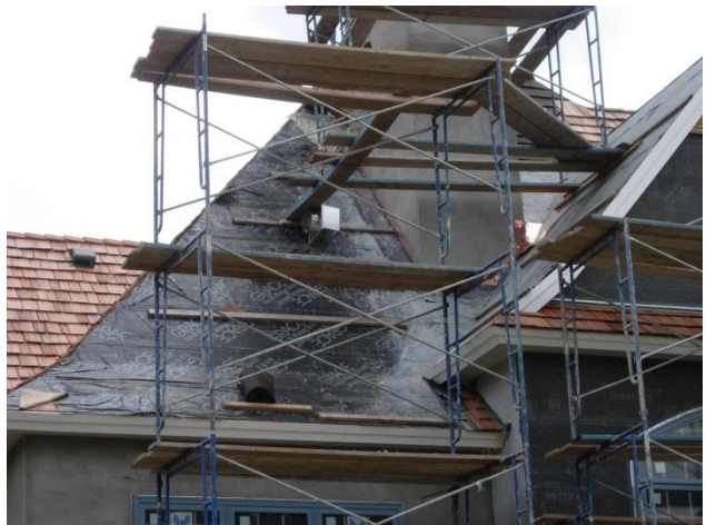
2 nd Inspection roofing
