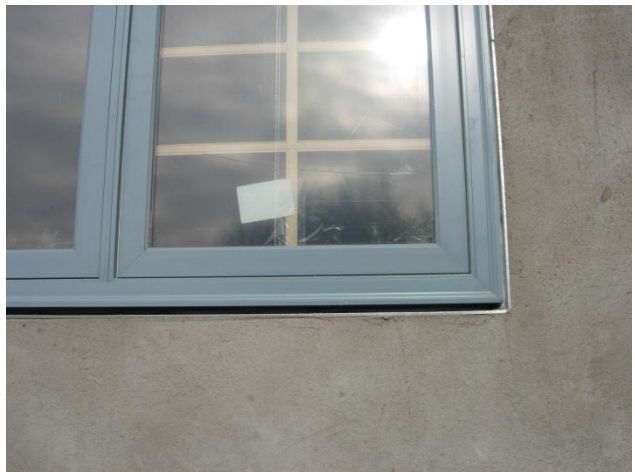
3 rd inspection caulking
