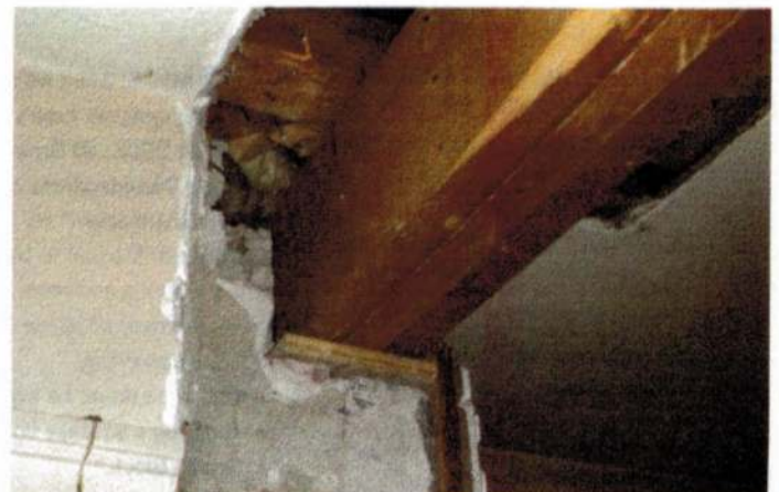
This photo shows a support beam that is inadequately supported and does not have adequate air gaps.
