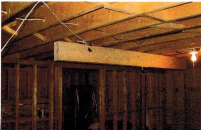
In this photo, the homeowner incorrectly added a post and beam to support additional live loads
