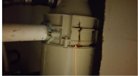
Cracked & leaking disposal
