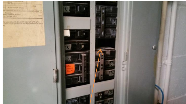
Missing circuit breaker knockouts
