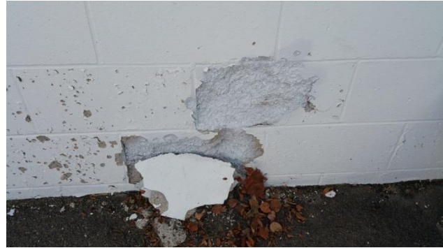
Deteriorated exterior blocks
