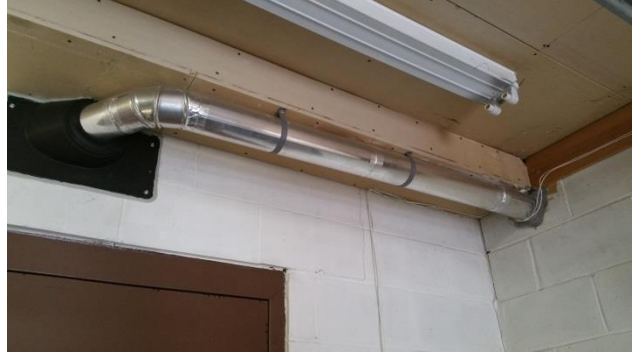
Unprotected dryer vent
