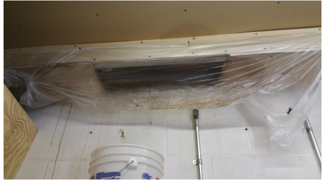
Water damaged ceiling plaster
