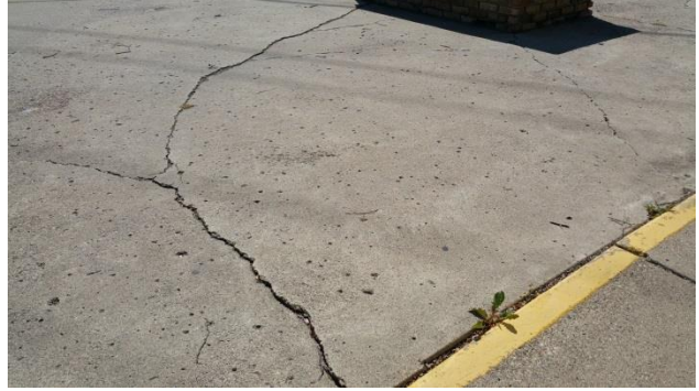
Cracked & uneven city sidewalk (assessment)
