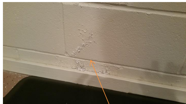
Water stained north wall
