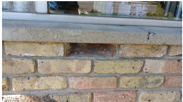
Deteriorated bricks
