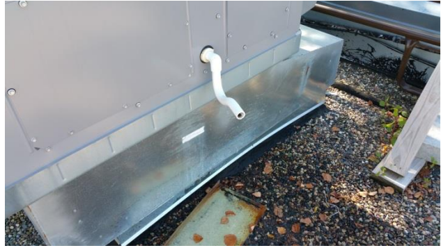
No condensate drain line
