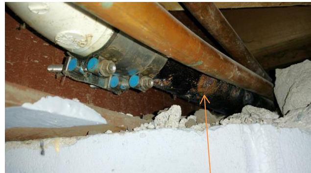
Corroded drain pipe
