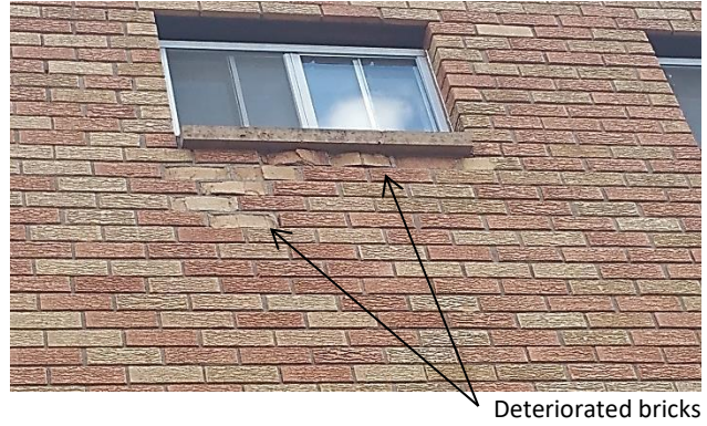
Deteriorated bricks
