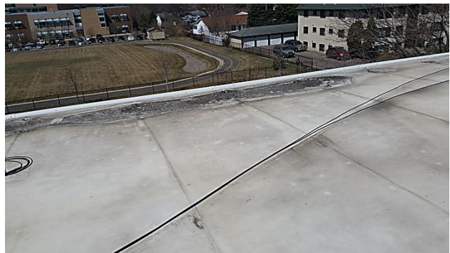
Buckled insulation
