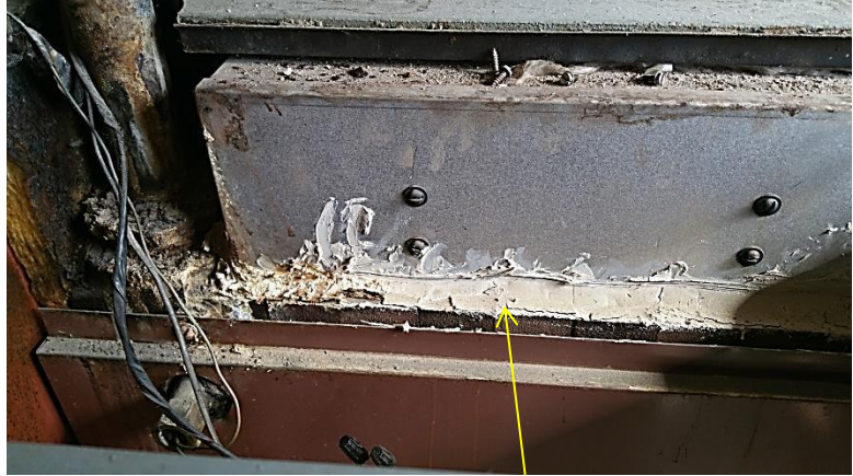
Temporary vent connection repair
