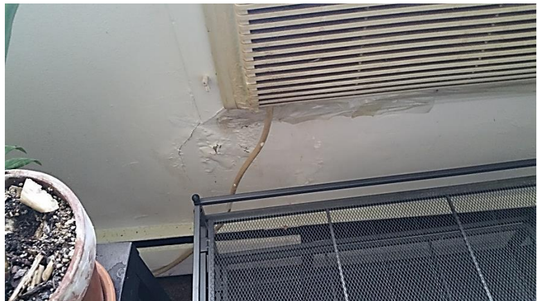
Damaged plaster at AC
