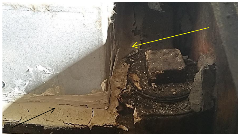
Temporary cast iron repairs
