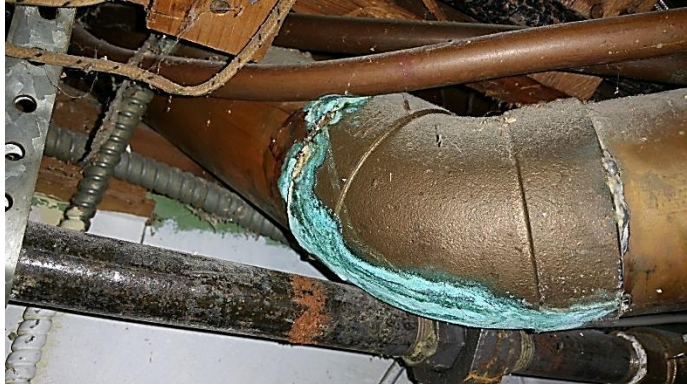
Leaking pipe
