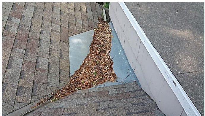
Restricted drainage – ice dams
