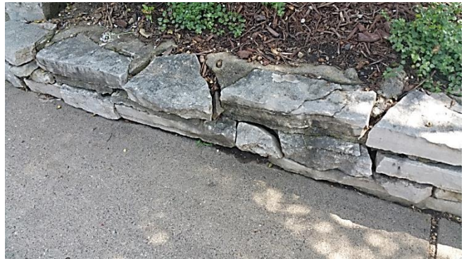
Retaining wall – loose stones
