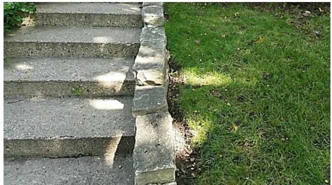
Retaining wall – tipped stones
