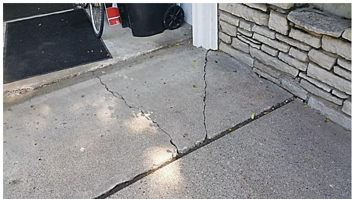
Cracked driveway apron
