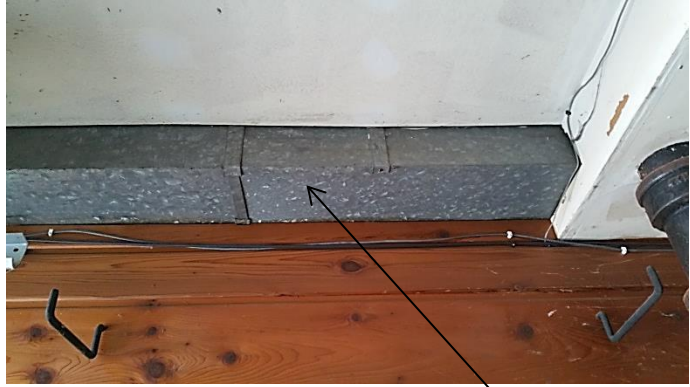
Unprotected duct
