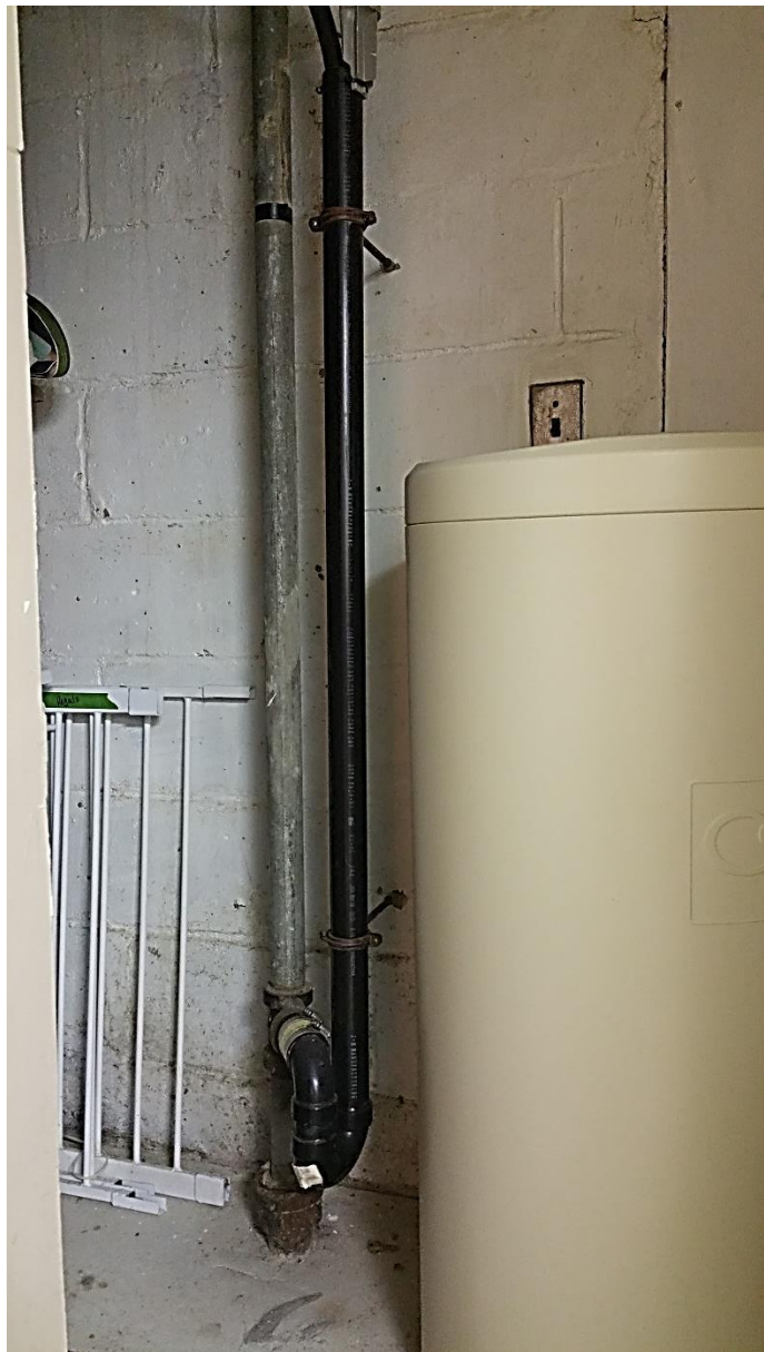
Standpipe too high
