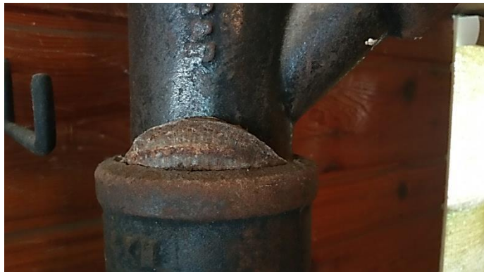
Loose lead connection
