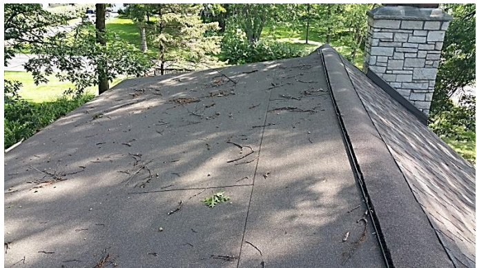
Low slope roof – no problems
