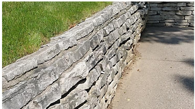
Retaining wall – bowed stones
