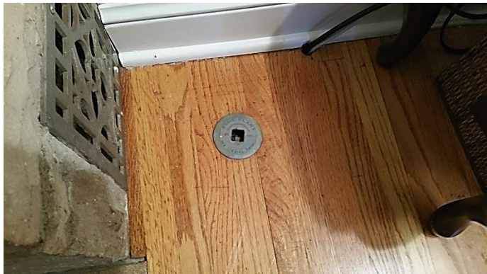
Fireplace gas shutoff
