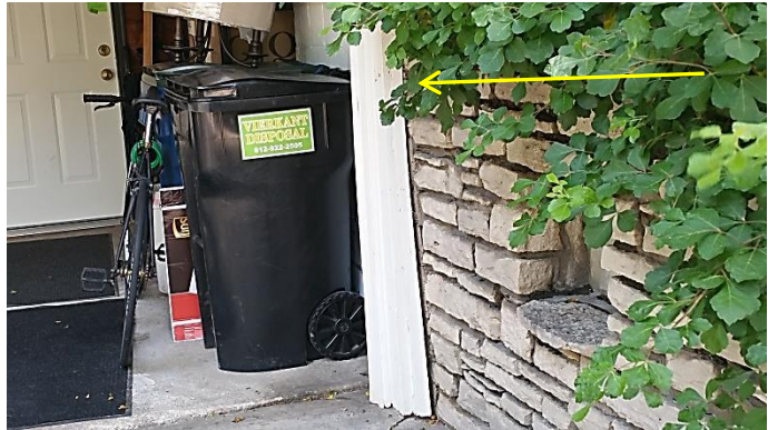
Retaining wall – tipped stones
