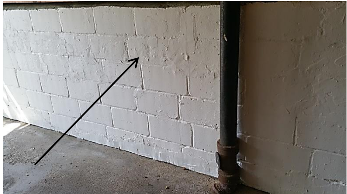
Patched blocks (water damaged)
