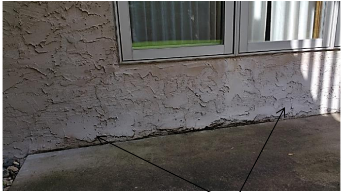
Water stained stucco
