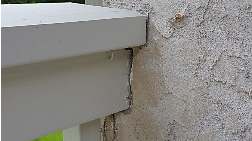
Guardrail in stucco (moisture intrusion)
