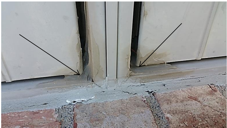
Excessive corner caulking (front only)
