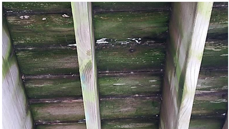
Decayed floor boards
