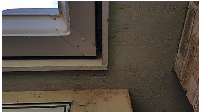
Water damaged soffit (front)
