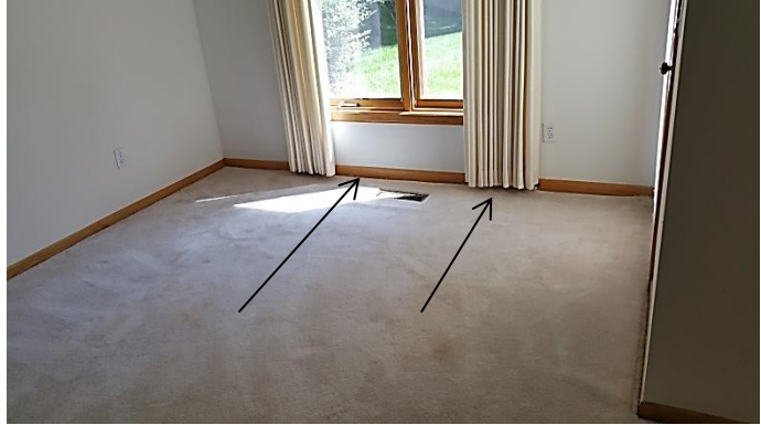
Water stained floor
