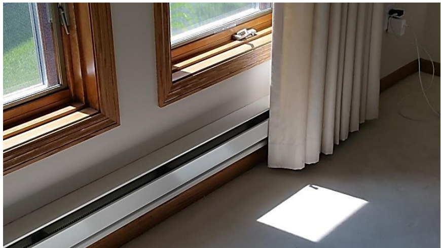
Drapes too close to heater
