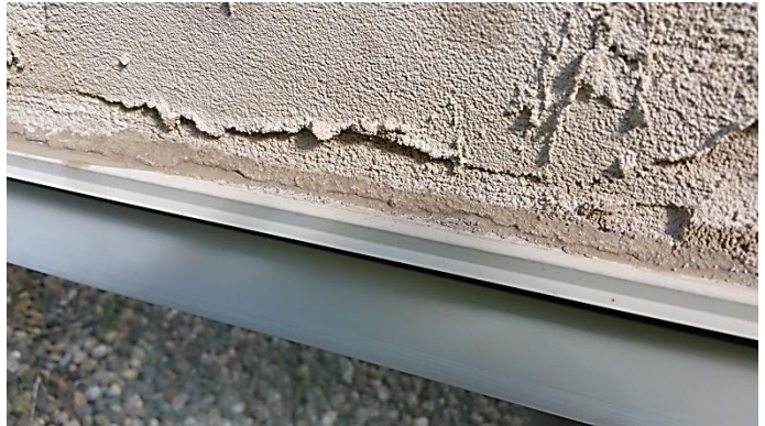
Caulked window top (traps moisture)
