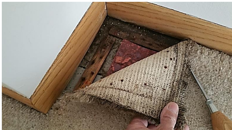
Water damaged floor
