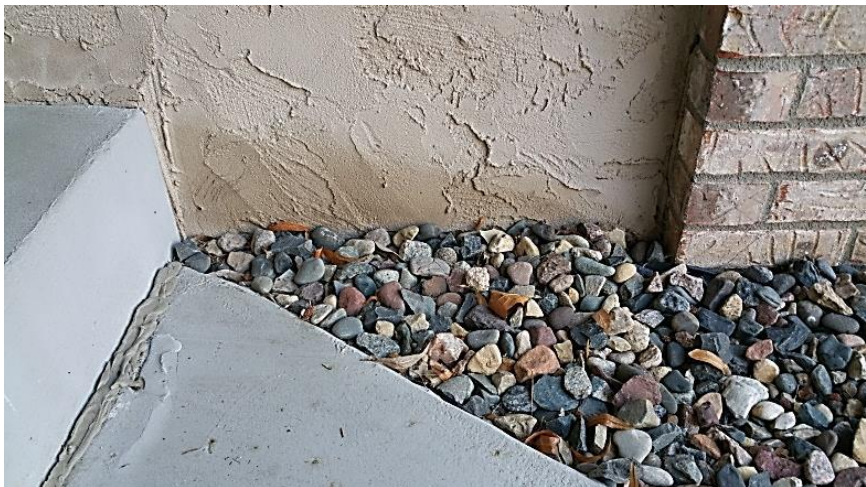
Stucco contacting earth
