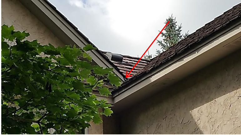
Restricted drainage (ice dam)
