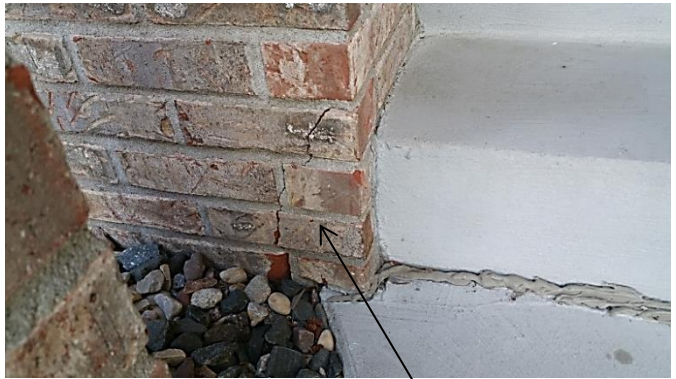
Cracked & settled bricks
