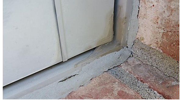
Excessive corner joint caulking (front only)
