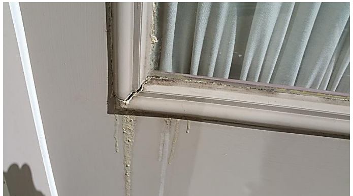
Cracked door trim
