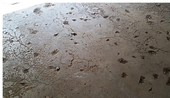
Pitted slab / deteriorated blocks
