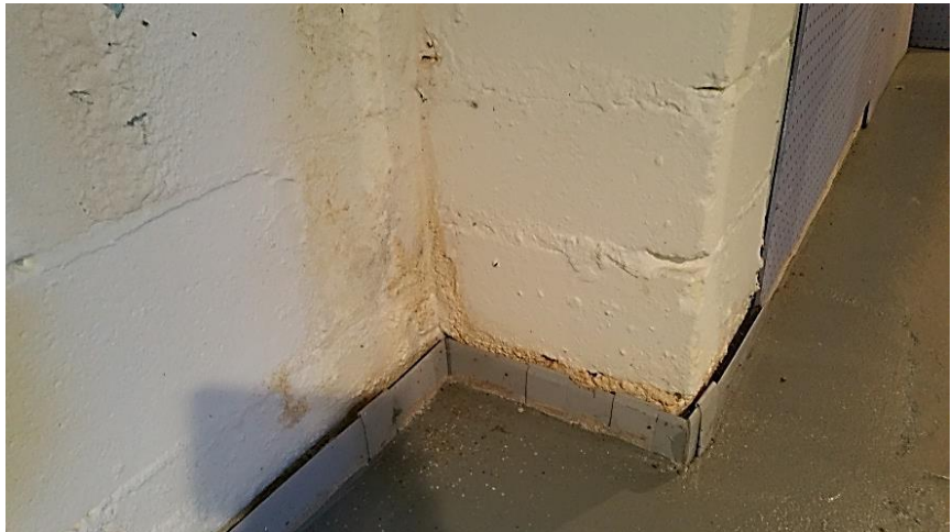
Water stained foundation
