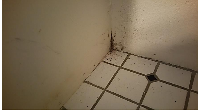
Water damaged wall behind shower
