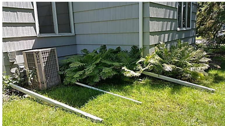
Flat grade (west side)
